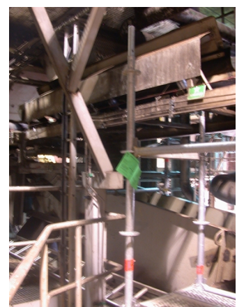
Scaffolding with a green label
