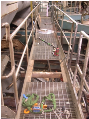
Grate removed to facilitate work
