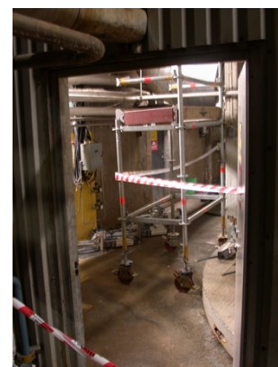
Temporary barrier for high-pressure spraying, soda recovery unit 4
